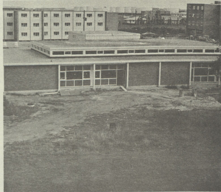
THE NEARLY-COMPLETED MSC Food Service is shown in the foreground. In the left background is Dahl Hall, with the men's dorm currently under construction to the right of Dahl Hall. This photograph was shot from the top of Livingston Lord Library by Mystic photographer George Wray.
