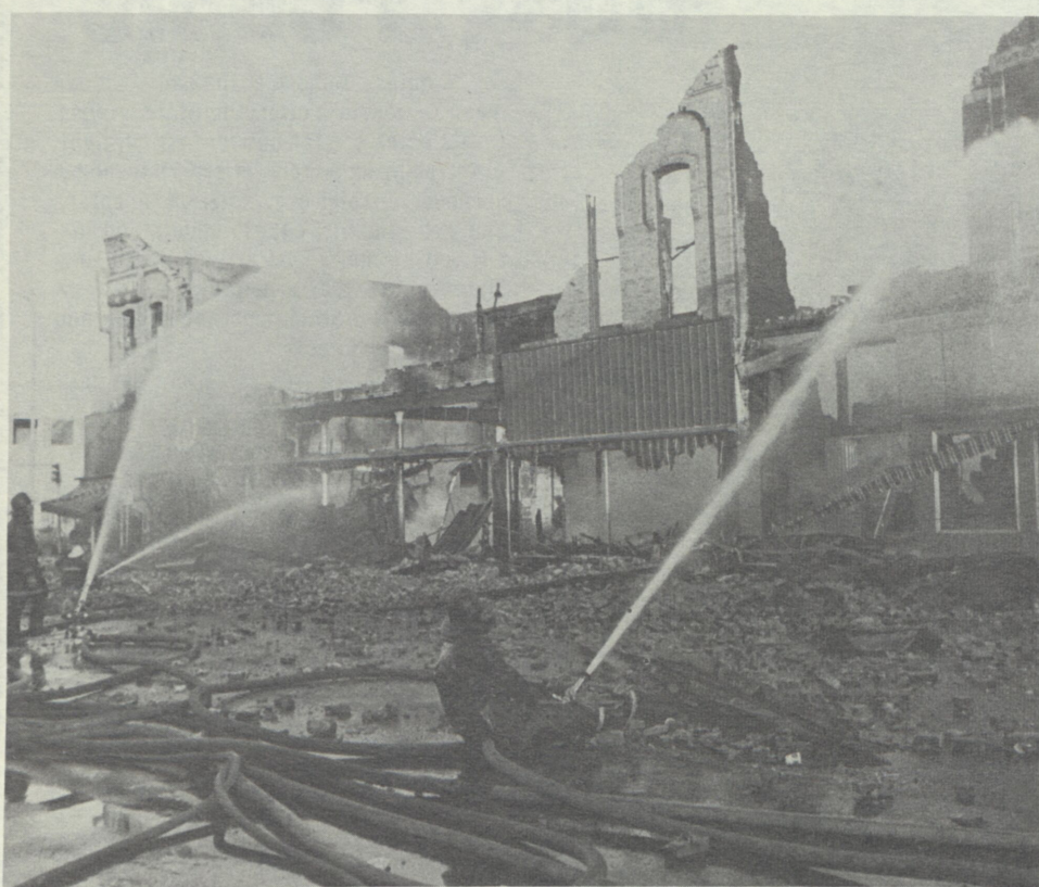
Firemen poured nearly 1,000,000 gallons of water on the Waterman's fire in Moorhead. Mystic photographer Erik took over 100 pictures of the fire which destroyed one half of the 600 block in Moorhead.
