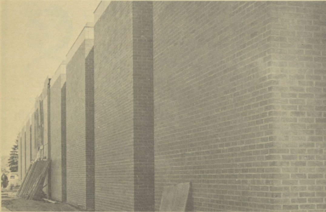
From the outside, the building looks nearly completed . . .
