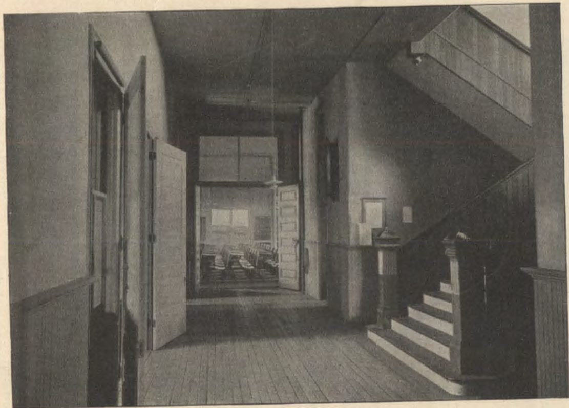
HALL, IN MAIN BUILDING.
