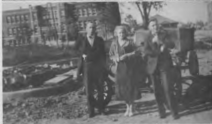
Majestic even in ruins was Old Main, as only the outlines of the three traditional arches stood the day after the fire of 1930. . . . Construction days began soon after the fire—toward the building of a larger and more modern educational center. . . . Smiling and happy are these three young students as they catch a glimpse of the new Moorhead Teachers College which was to be. . . . DR. G. L. GOSSLEE, resident director of the Teachers College, to whom belongs some of the credit for the present-day institution.
