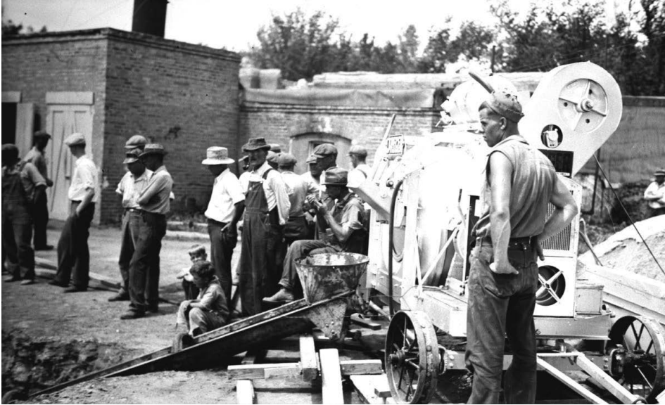
Construction begins on the new buildings.
