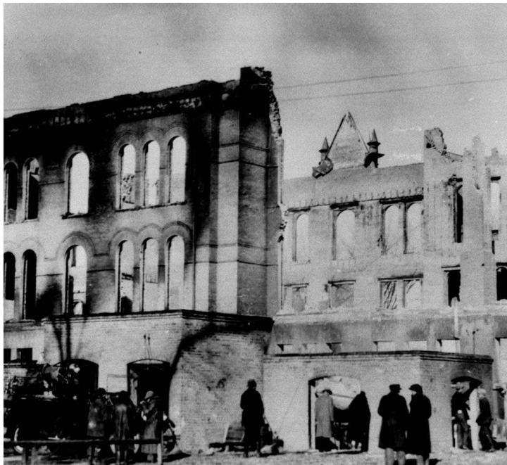
Salvage work begins on the power plant, while classes are held in Weld, the dormitories, and nearby homes.
