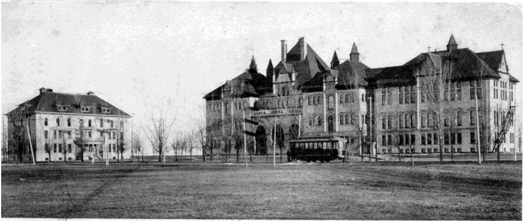
The Moorhead city trolley ran a regular route out to the campus from the late 1890s until it was replaced by more modern street cars in the 1920s. During the depression of the 1930s, the street rail closed down, after the local electric company cut its traditional discount to the Moorhead and Fargo city governments. When World War II came in 1941, the rails from the street railway were finally removed from the streets and sold for scrap. Above – Old Main and Wheeler Hall, the sole dormitory in the early 1900s.
